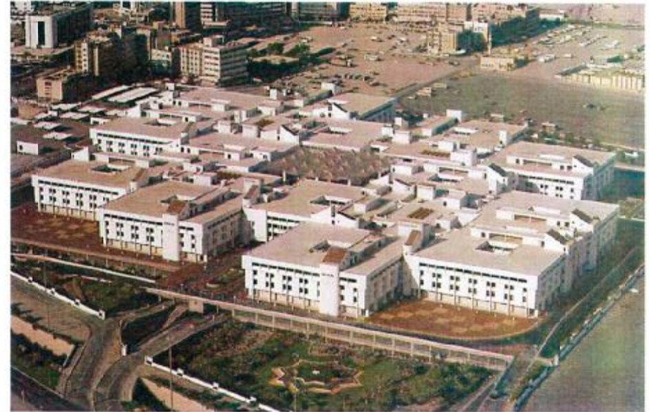
Ministries Complex Buildings, Kuwait
