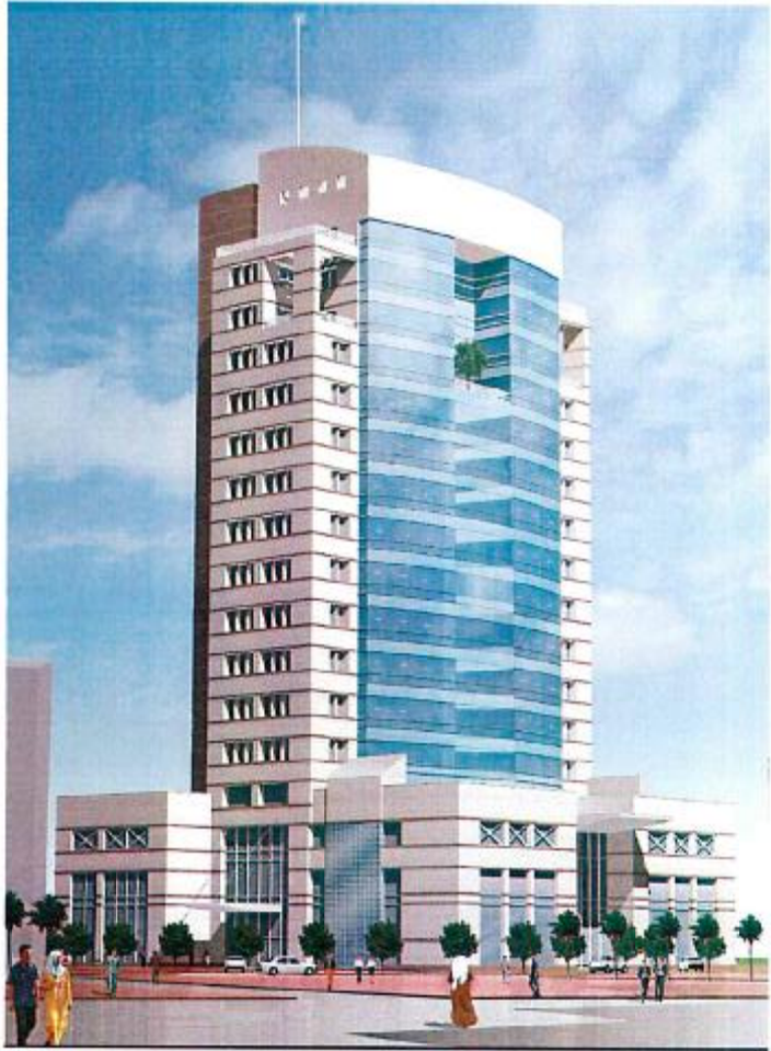
HAWALLY EDUCATIONAL BUILDING-247
