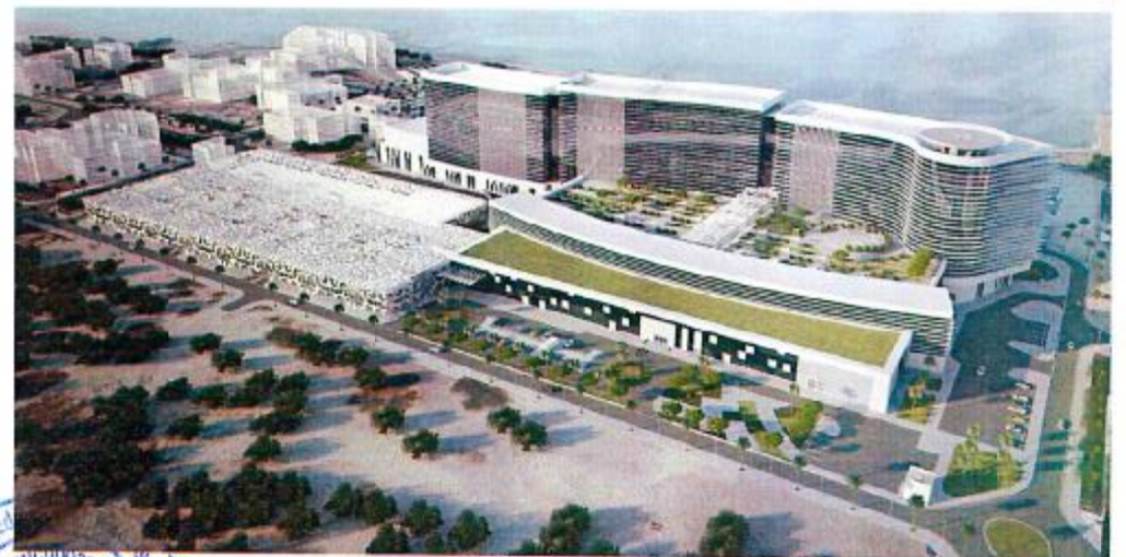
New Al Sabah Hospital
