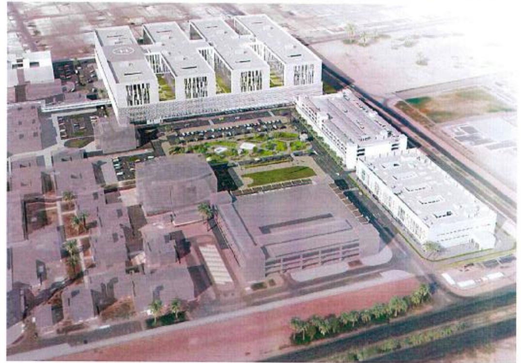
Expansion of Farwaniya Main Hospital
